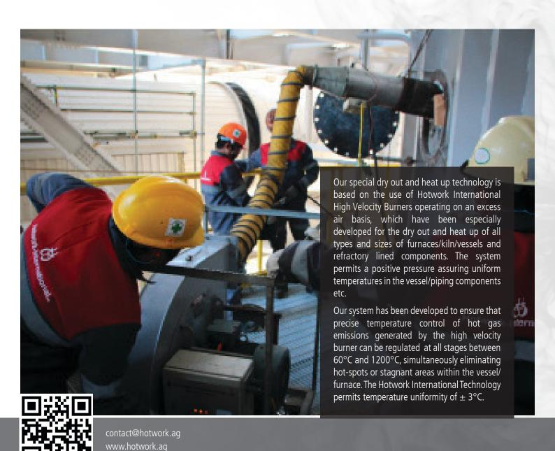
**Hotwork International** provides dry out service for the refractory lining as well as heat treatment service for welded steel components on full power generation units, such as power boilers, CFB boiler, Heat recovery steam generator (HRSG), incineration plants, furnaces, ash hoppers, ducting components, cyclones, burners, floors, flues, target walls, chimneys, as well as any kind of boiler and component.
